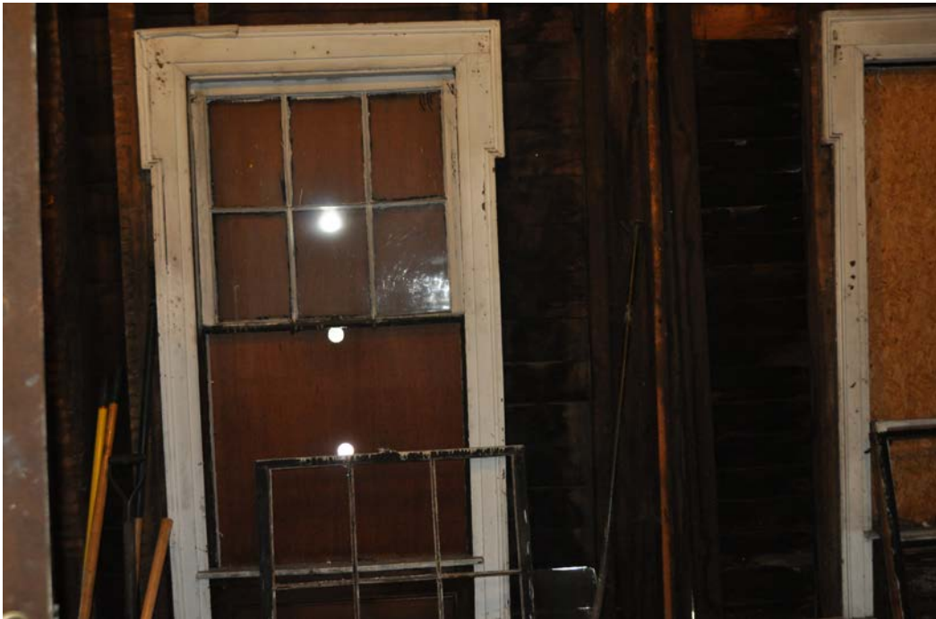
Picture #3 shows one of the 3 windows in the Dining Room. The window trim design is called "dog-eared" This picture also shows where I am removing the old sashes to be restored.
