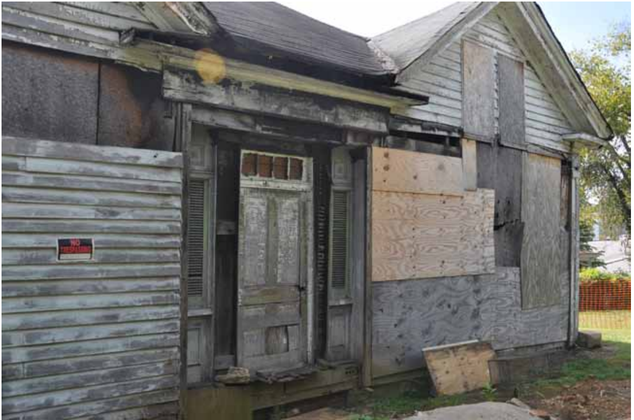
Picture #2 is a current view of the back side of the house. I have not done any work on it. There are two windows that were removed when the addition was put on back in the early 1920s that will have to be built and installed.
